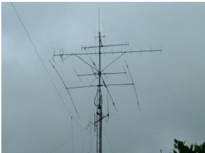
**VHF and HF Short Wave beams used to communicate around the UK and the rest of the world.**
